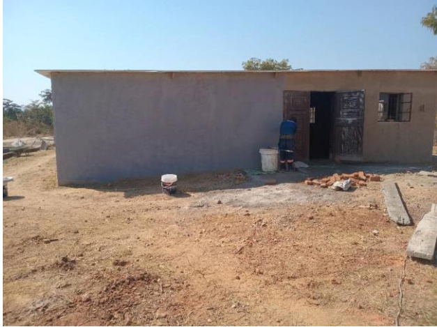
Figure 2 - Grain storage / Milling Room entrance
